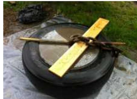
950mm dia tyre being filled with concrete. Note heavy chain secured with steel rod in the middle of the concrete to ensure secure attachment. This weighs about 250 kg in sea water so slightly less than a standard train wheel.
